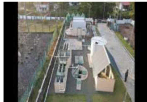
1 MLD CSTP at Padanappalam, Kannur
